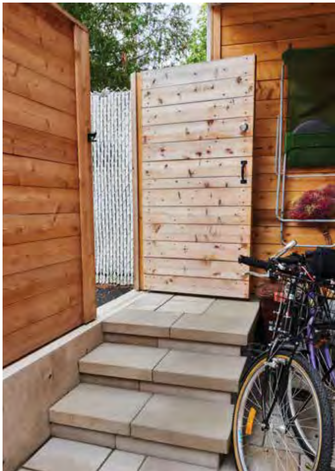
This small storage area becomes a thing of beauty, paved with Unilock Beacon Hill™ Smooth and Universal Coping treads.
